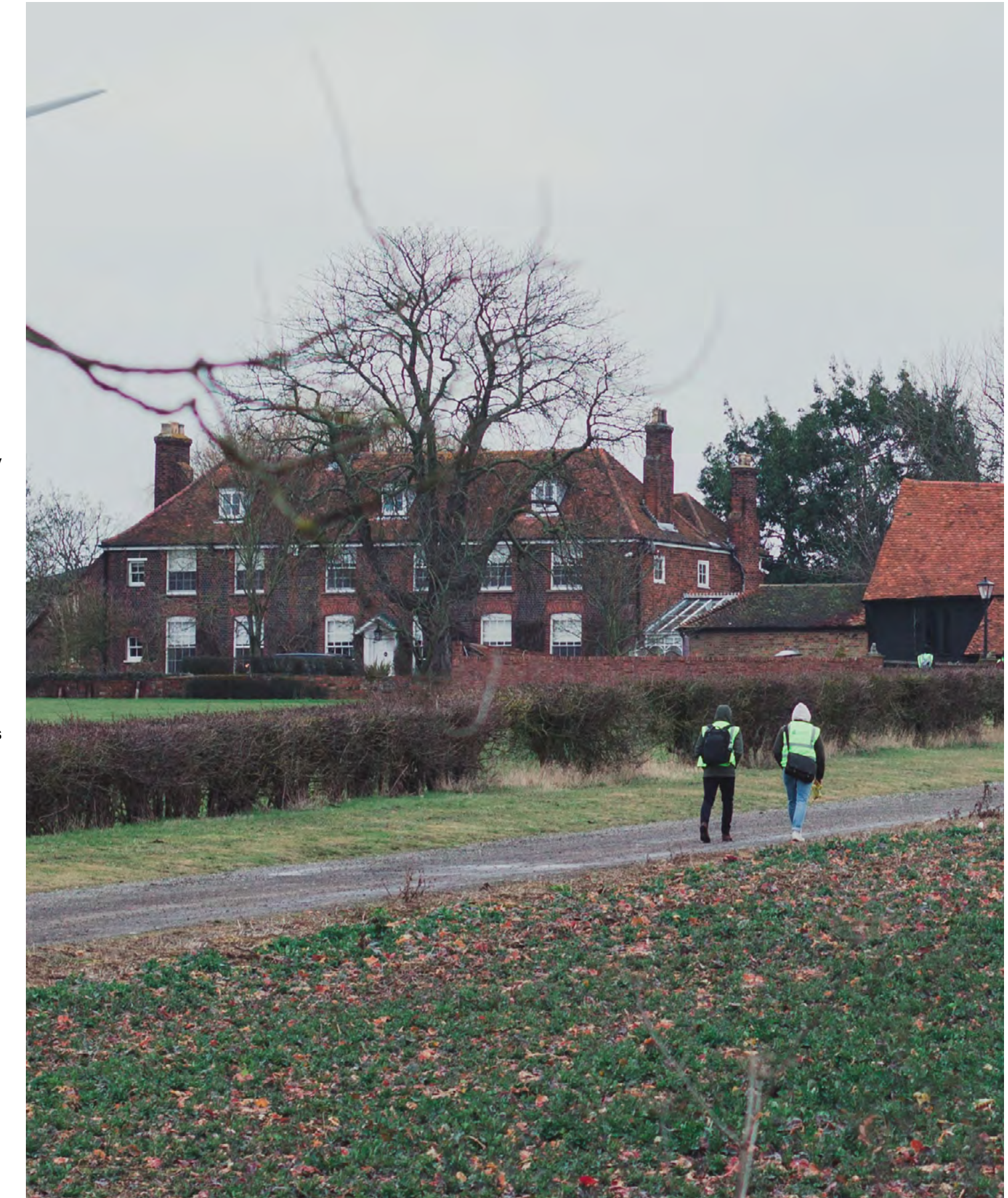
Figure 2. Image of the Grade II listed Dunton Hills Farmstead
