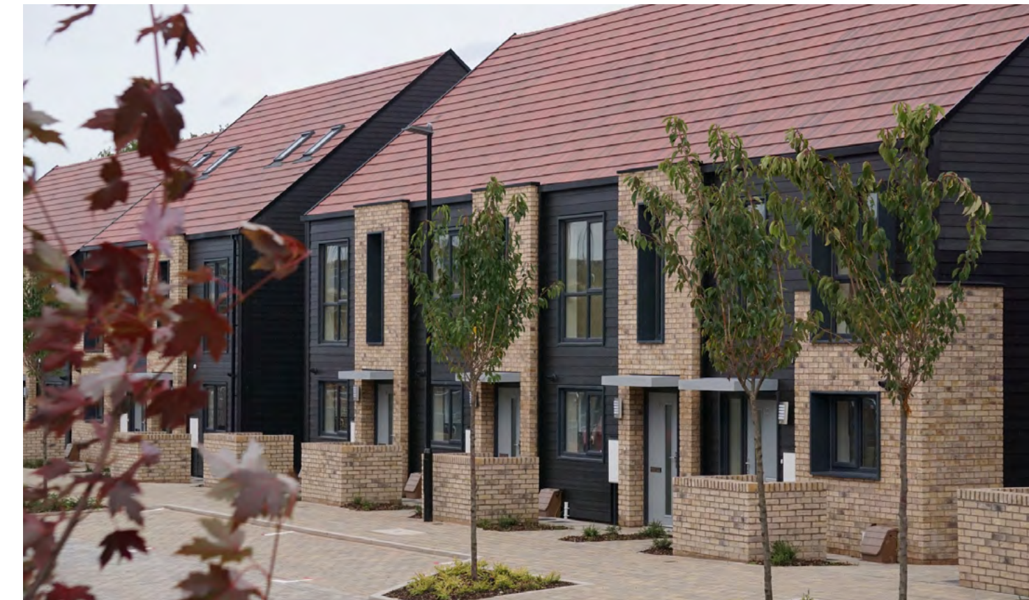
Figure 40. Welcoming and accessible entrances
