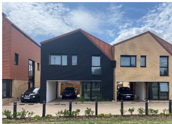
ITP – Fryerns (Basildon). Showing on plot parking incorporated into driveways and undercroft.
