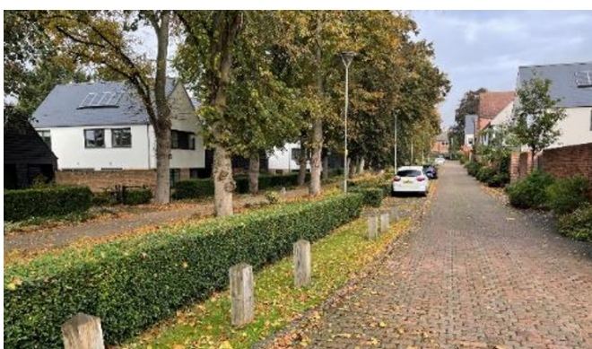
ITP – The Avenue (Saffron Walden). Showing landscaping to deter on-street parking outside of dedicated bays.
