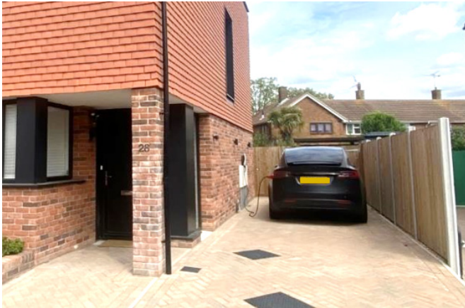
Figure 4-1: Residential on-plot EV charging 20
