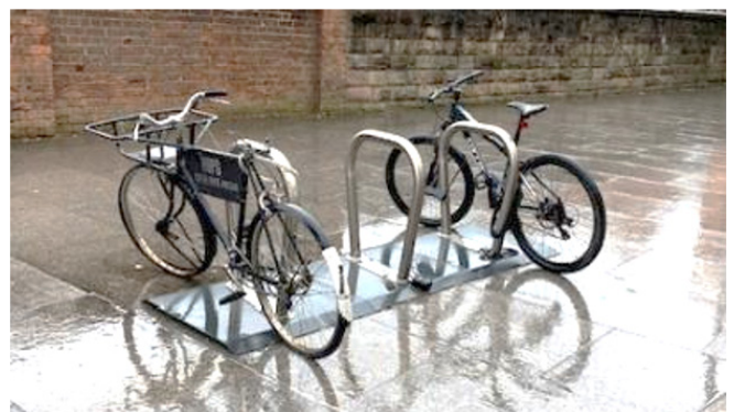
Figure 3-4: Recommended arrangements for Sheffield stand provision
