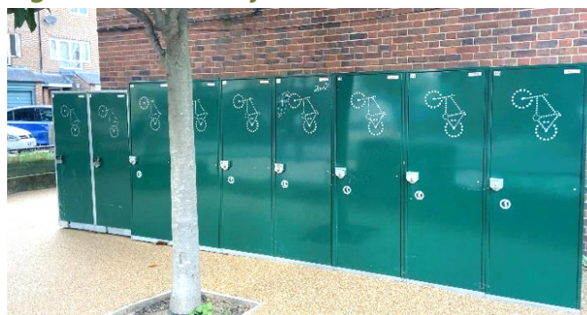
Figure 3-9: Metal cycle lockers 14
